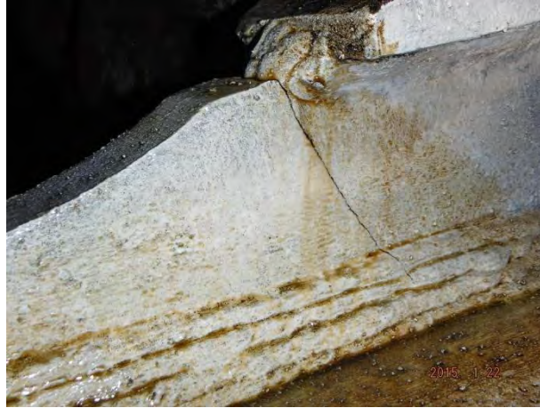
Fig.12: Example of close-up image of a crack. The crack is in the foreground, in sharp focus and neither over- nor under-exposed. The upper left of the image is however underexposed (pitch dark) and out of focus (blurry).
