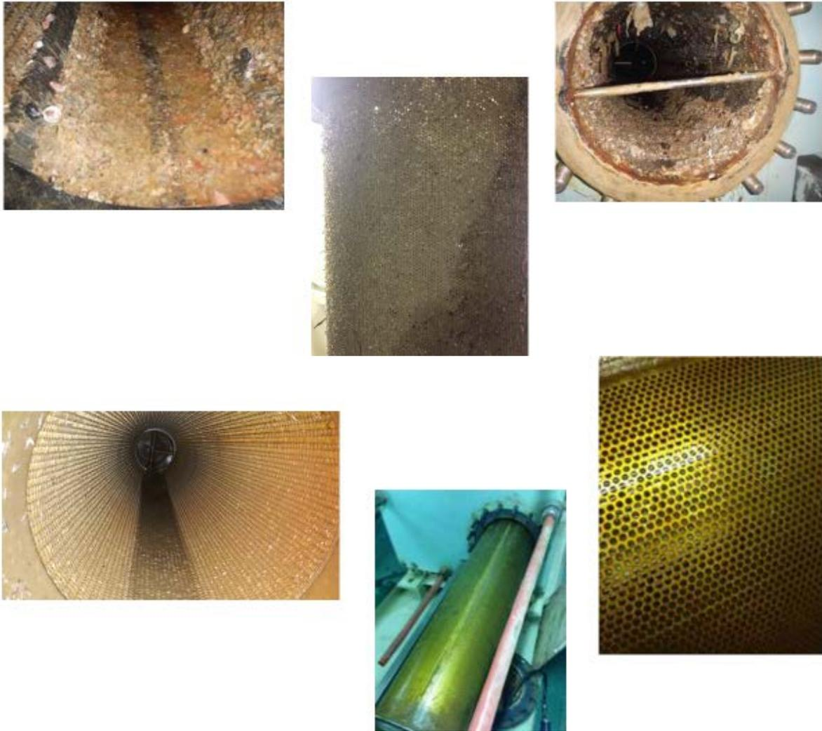
Fig.6: Low-temperature cooler on 13000 TEU containership without (top) and with (bottom) ultrasound protection after 13 months trading Europe / Fareast Asia
